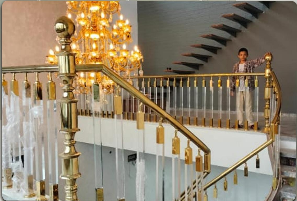
**Acrylic railing designs offer a modern and stylish alternative to traditional glass railings. Made from high-quality acrylic sheets, these railings provide excellent transparency with a lightweight yet strong structure. Acrylic railings are ideal for staircases, balconies, terraces, and indoor spaces where a clean, contemporary look is required..**
